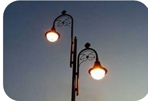
Completion of a Small Cell Licence Agreement to provide controlled access to our street assets to MNOs
